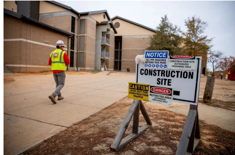
Tim Gouger, USACE Omaha District, Rapid Response Technical Center of Expertise Program Manager, on site at one of the eight newly renovated volunteer army (VOLAR) barracks at Fort Liberty.
