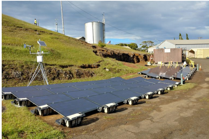
Photo 3: Lightweight solar panels on Mt. Koke'e, Hawaii demonstrate rapidly-deployable, off-grid energy technologies for increased mission energy resiliency in remote locations.
